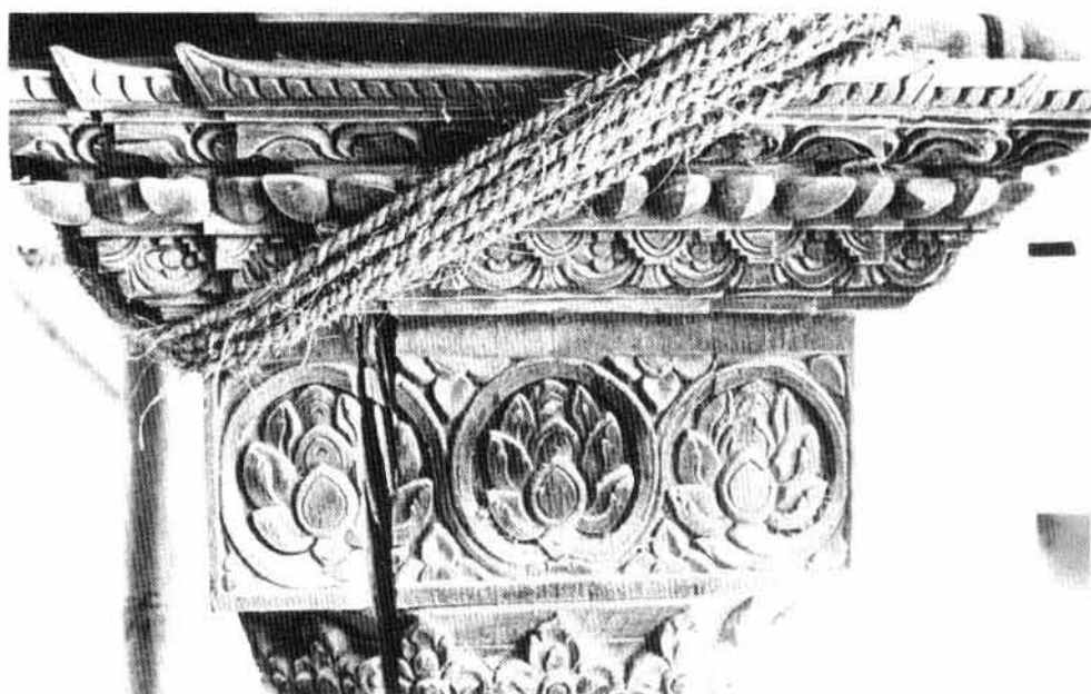
Varying carved floral motifs just below the capitals of arcade-level pillars, two pillars on north elevation. The vertical cracks are typical of historical timbers in Nepal which are never seasoned before carving and installation.
